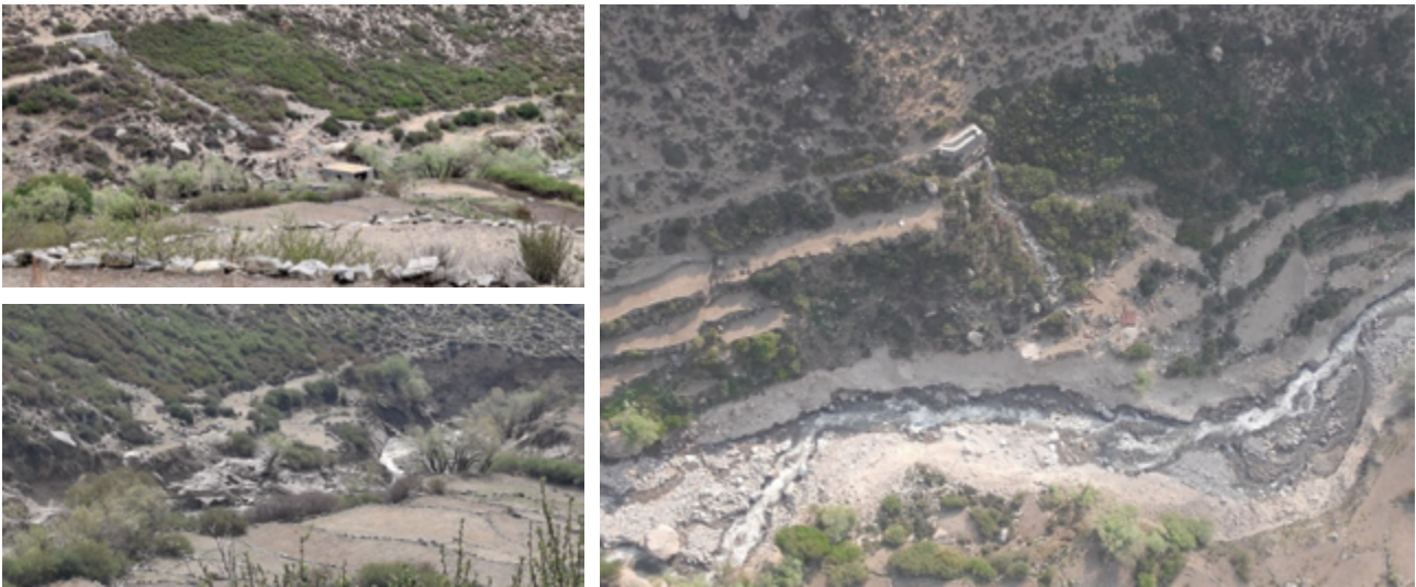
Figure 18: Pre- and post-event field photographs show the 15 kW hydropower station, which was under construction, completely washed out by the flood. (Left photo by Penpa Dhondup, Ward Member of Limi Rural Municipality; Right photo by Sudan Bikash Maharjan).
