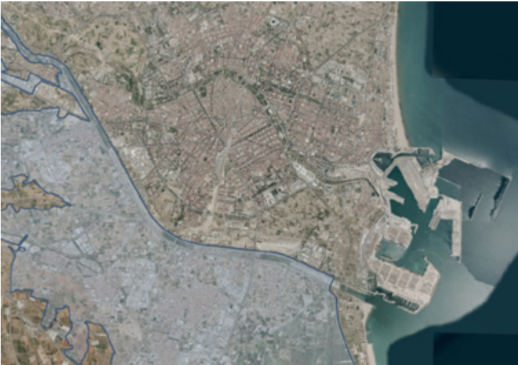
Figure 19: South Plan (Plan Sur) infrastructure also acted as an unintended barrier for certain flood runoffs in the southern flooded area (Saleta Ravine)
