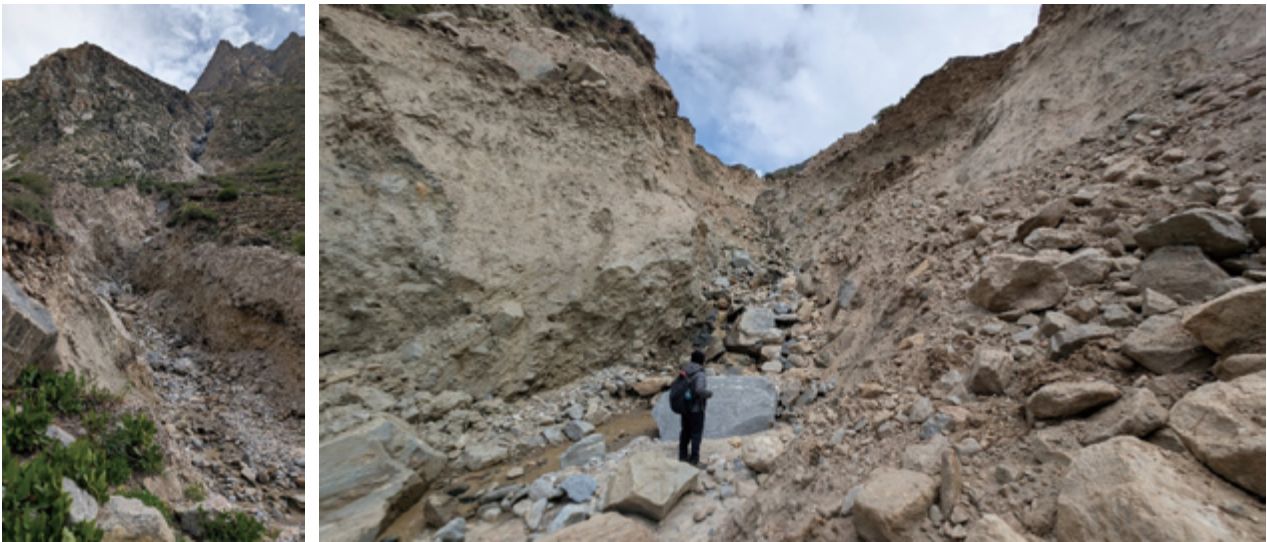
Figure 17: Field photographs showing deep vertical incision and erosion on the talus fan deposits, along with progressive bank failures to the east of Til village. (photo by Sudan Bikash Maharjan)
