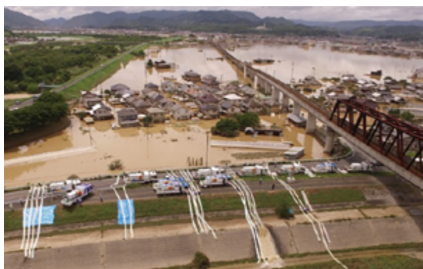
Figure 3. Emergency Drainage Using a Drainage Pump Truck
