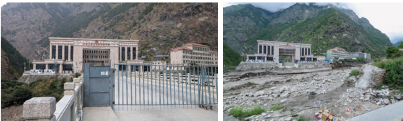
Figure 22: Before (November, 2024) and after (9 July 2025) photographs showing the Nepal-China Friendship bridge was completely wash out by GLOF. (Photo by Sudan Bikash Maharjan{left} and Online{right})
