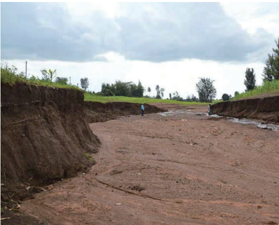
Figure 12: Deep gully erosion caused by water from the Solai Killer Dam
