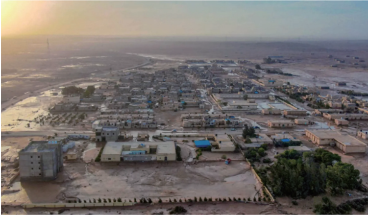
Figure 7: General view of flood water covering area in Almkheley town (Source: Libya Al-Hadath / Teuters)
