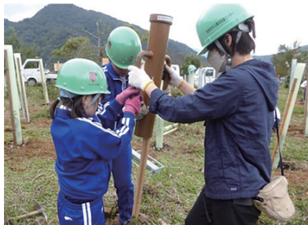
Picture-7 Installing posts to protect against winter snow.
