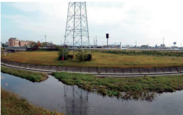
Fig. 18 Itonuki River, before improvement
