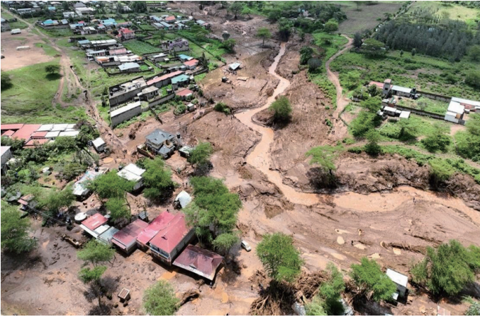
Figure 33: View of damaged houses after heavy flash floods in Mai Mahiu, Kenya.
