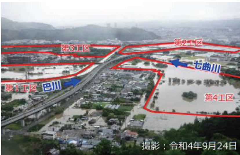
Fig. 8 Asahata Flood Control Basin storing floodwater in the 2022 flood (Source: Shizuoka Prefecture)
