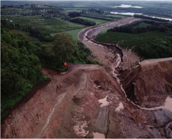
Figure 13: An aerial view of Solai dam
