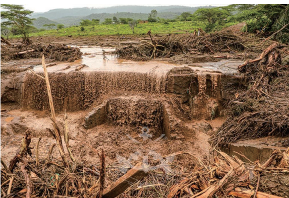
Figure 35: Destroyed road crossing at Mai Mahiu
