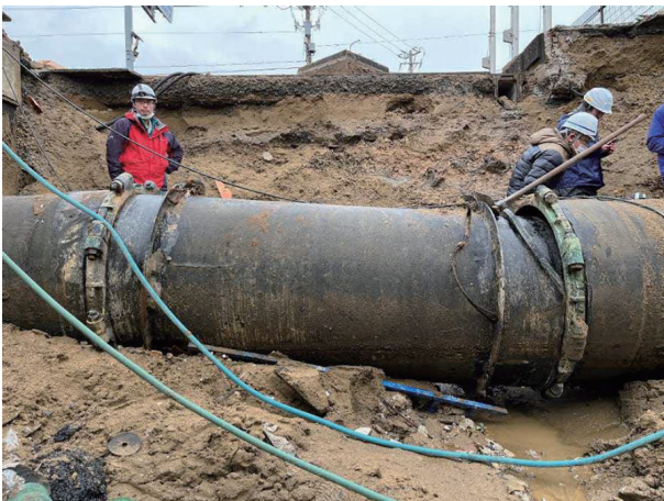
Figure 1. Damage to Vital Facilities in Water and Sewerage Systems (left: water supply pipe; right: pressure pipe directly connected to the treatment plant)
