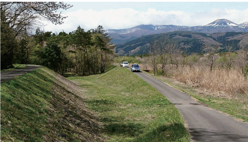
Fig. 4 Open levee system in front of the flood protection forest
