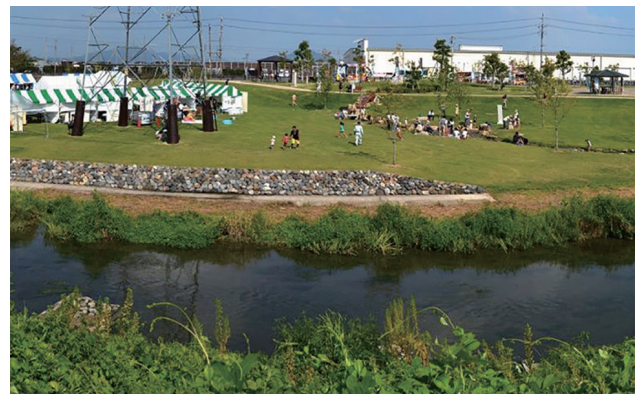
Fig. 19 Itonuki River, after completion
