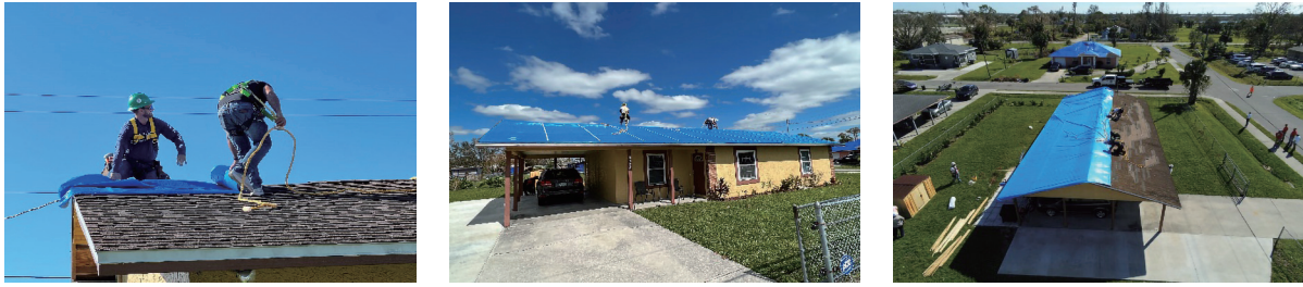
Figure 11. Contractors install blue reinforced plastic sheeting as temporary roofing as part of Operation Blue Roof until more permanent repairs can be made. (Brigida Sanchez and UAS Team - USACE Jacksonville District)
