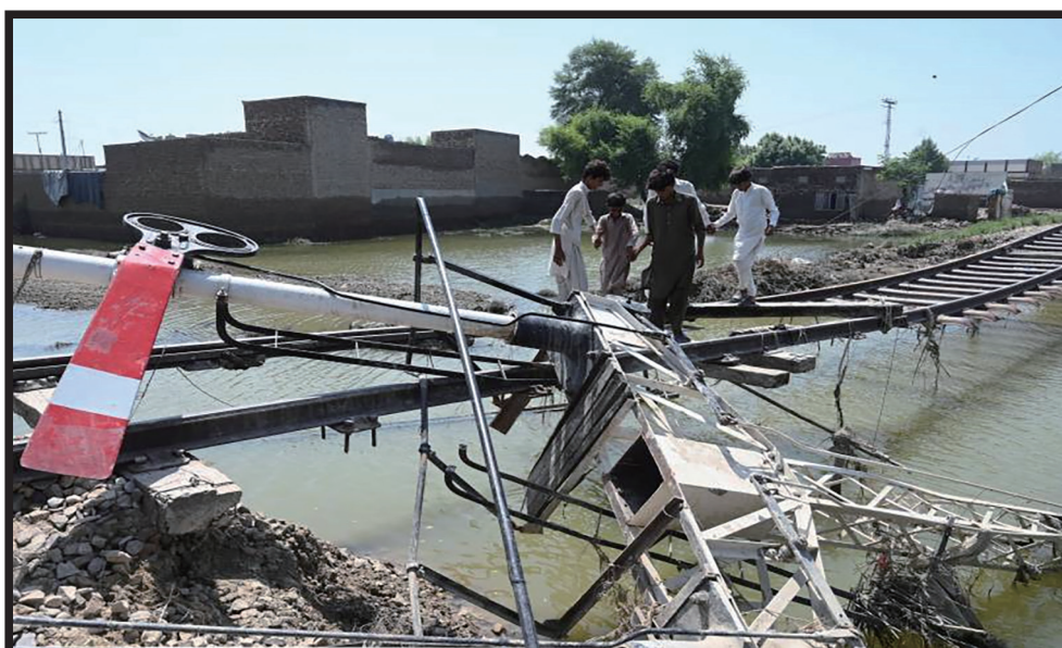
Damaged Railway Line – Embankment Washed away under the Railway Track
