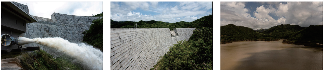
Figure 6. The Portuguese and Cerrillos Dams were able to hold approximately 20 million cubic meters of water combined during Hurricane Fiona. This volume of water would have flooded almost the entire urban area downstream of the dams. Rough preliminary estimates for the prevention of flood damages from both dams and associated channels are over $100 million. More importantly, thousands of priceless lives were saved, (Brigida Sanchez - USACE Jacksonville District)
