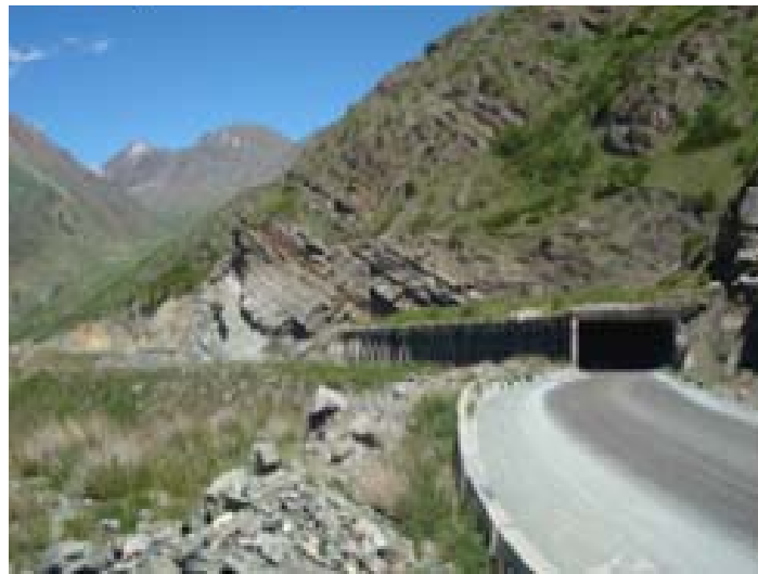
Gallenes protecting the road from landslides
